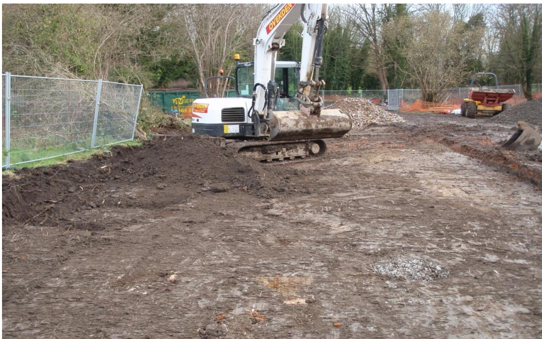
Plate 3 The site showing Phase 1 reduction of site of Area 1 (looking east)
