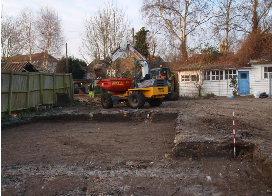
Plate 6 Phase 1 site reduction Area 2 (looking southwest)
