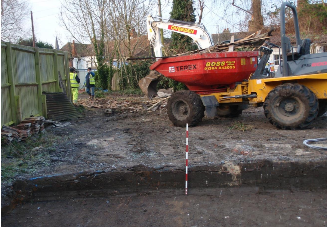
Plate 8 Phase 1 site reduction Area 2 close-up (looking southwest)
