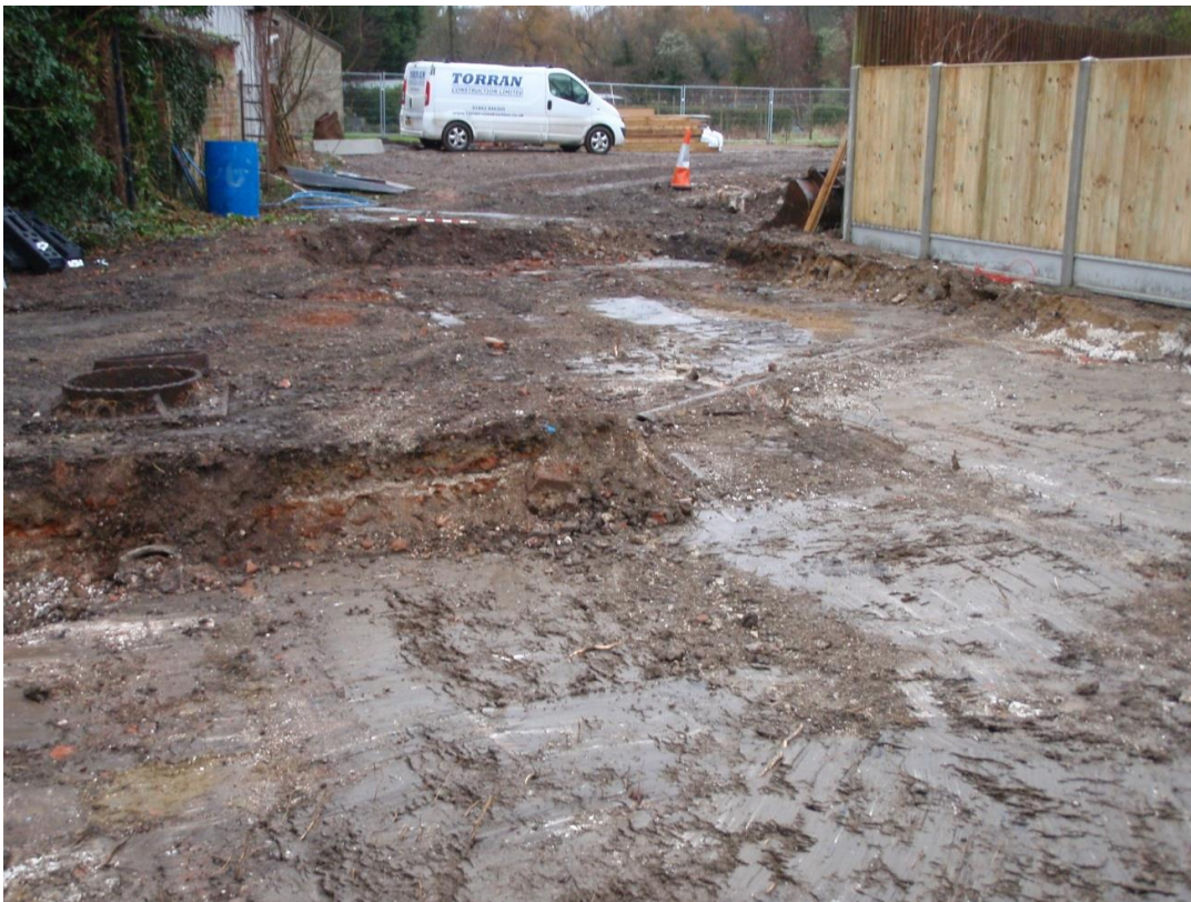
Plate 9 Phase 1 site reduction Area 3 (looking north)
