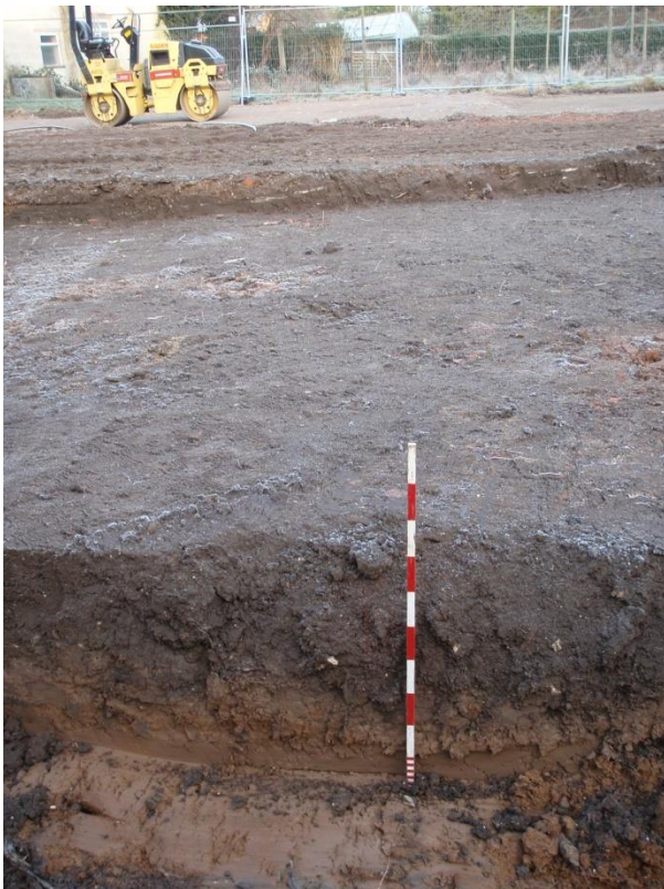
Plate 11. Phases 1 & 2 site reduction within the northern extent of Area 3 (looking north) – note Area 1 during Type 2 compaction in the background.
