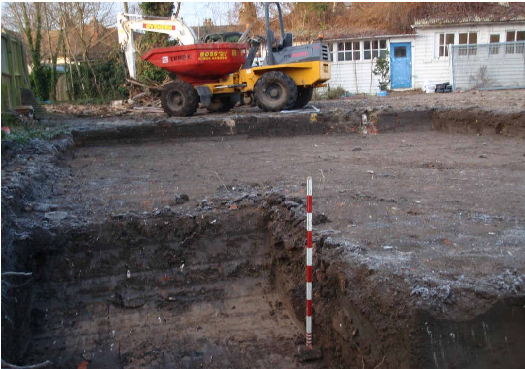
Plate 7 Area 2 during Phase 2 site reduction (looking southwest)
