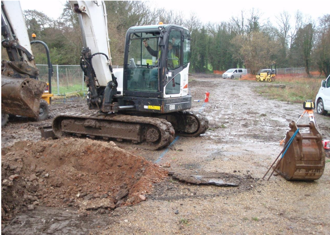
Plate 2 General view of the northern (Area 1) area of the site (looking north-east) at the start of Phase 1 excavation
